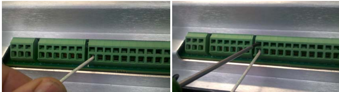
Figure 2-1. Installation of Wiring into Terminal
